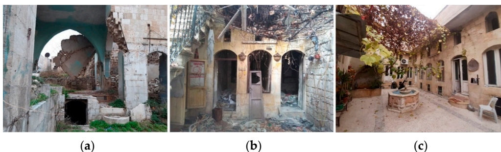
Figure 3. A house that was completely destroyed, Cadastral number 558 (a); a house that was severely damaged, Cadastral number 568 (b); a house that was not affected, Cadastral number 576 (c); Al-Jalloum neighborhood, Old Aleppo, winter 2020, Source: C. Kousa and students' work.
