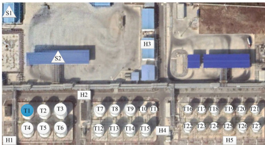
Fig. 4.4 Chemical storage facility considered in the case study (Chen et al. [1])
