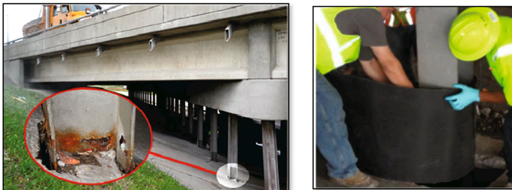
Fig. 15. One of the 49 corrosion damaged piles in I-70/I-270 Interchange (USA) that were repaired with wrapping FRP technique [98].
