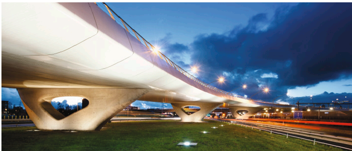
Fig. 1. Fly-over Waarderpolder bridge in Netherlands with FRP edge elements [10]. A single column fitting image.
