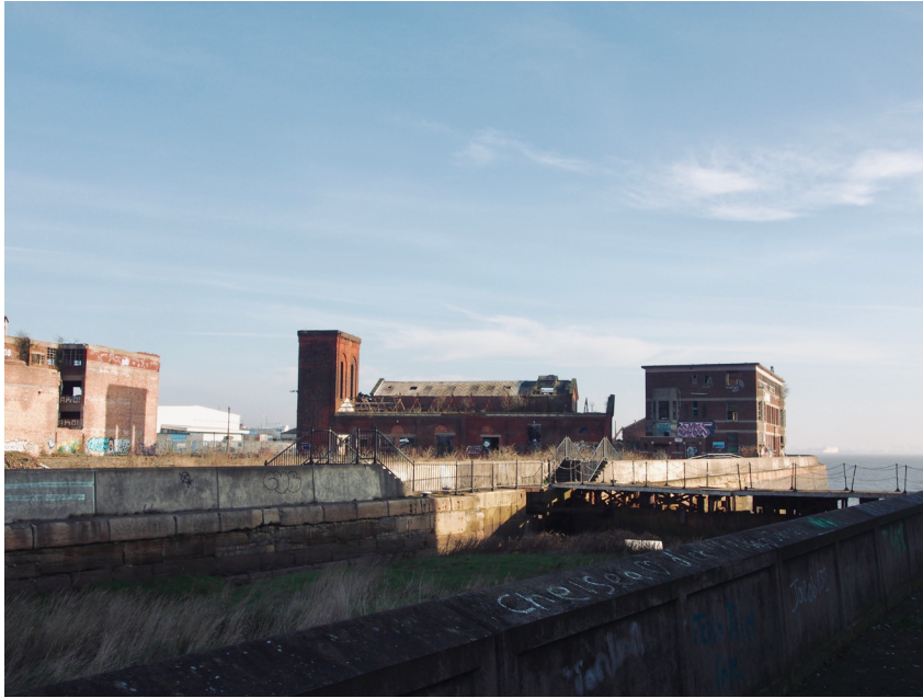
FIG. 13 Vandalized condition of St Andrew's remaining Lord Line building (left) and Grade II Listed Pump House (right) and lock gate (front), original photo by author, 2020.
