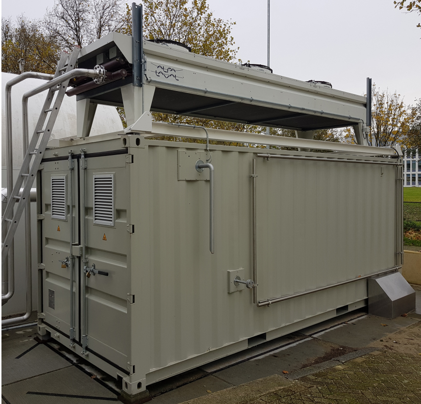
Figure 5.10: A photograph of the WTE 10-10-400-2-BHTT electric oil heater mounted in a container outside the Propulsion and Power Lab at Delft University of Technology. The aircoolers are located on top of the container.
