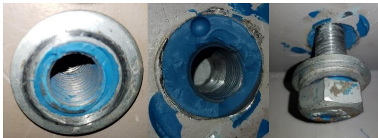
Fig. 5. Injected bolt holes
