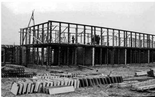
Figures 4.4.122 and 123: houses under construction, using the small element building system; 1950 interior. Gemeente Archief Amsterdam.
