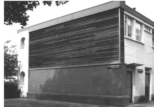
Figures 4.4.124 and 125: the rear of the houses with plastic window frames and the end elevation with brickwork and wooden cladding, 1987. H. Zijlstra 2002.
