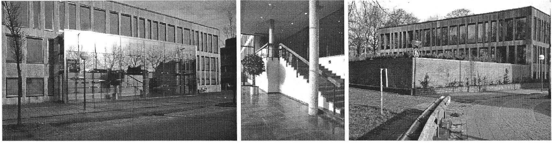
Fig. 11. The new entrance (exterior) of 1999. From: H. Zijlstra, 2002.
