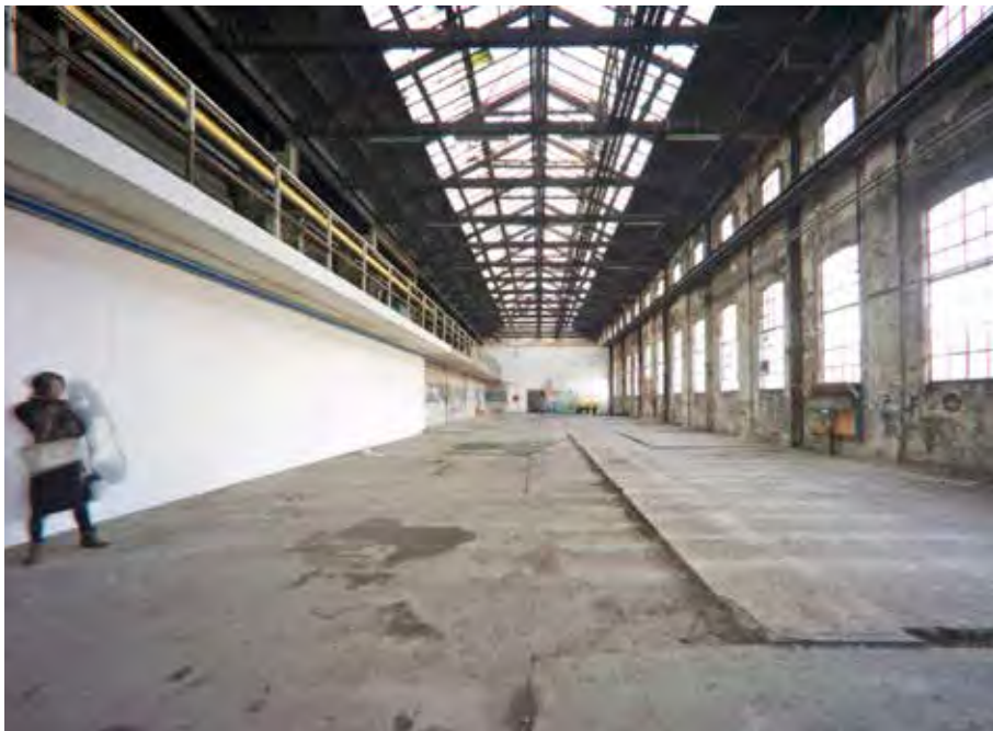
Figure 160 Van Gendhallen in Amsterdam's Oostenburgereiland.
