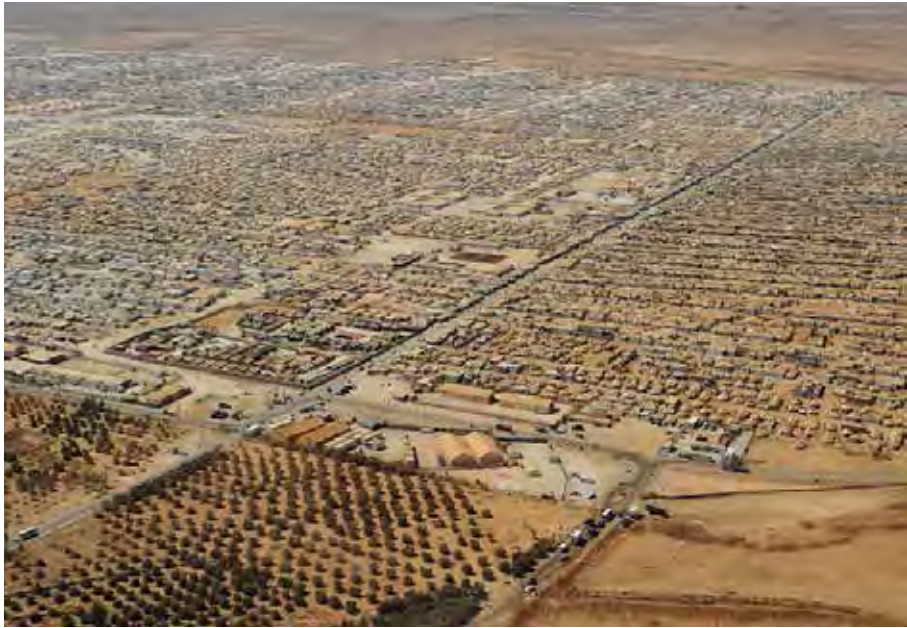
Figure 15 Aerial view of Al Zaatari.
