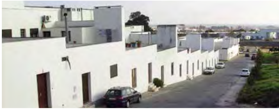
Figure 4 Malagueira Settlement before residents' adaptations.
