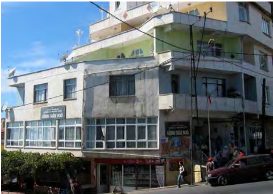
Figure 40 Public facility in Gulensu: the health clinic.
