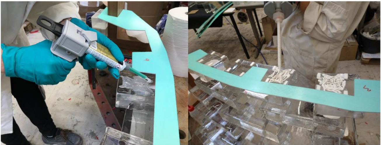
Fig. 17 Application of the 3M™ DP610 adhesive (left) and DOWSIL Experimental Fast Curing adhesive (right) during the construction of the prototype. Double-sided tape of clear (left) or white (right) colour were used to fix the bricks in place until the glue had hardened and to
