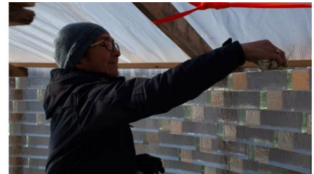
2. Bricks of the bottom layer are cleaned
