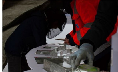
3. Bricks are placed into position using a CNC cut plastic jig.
