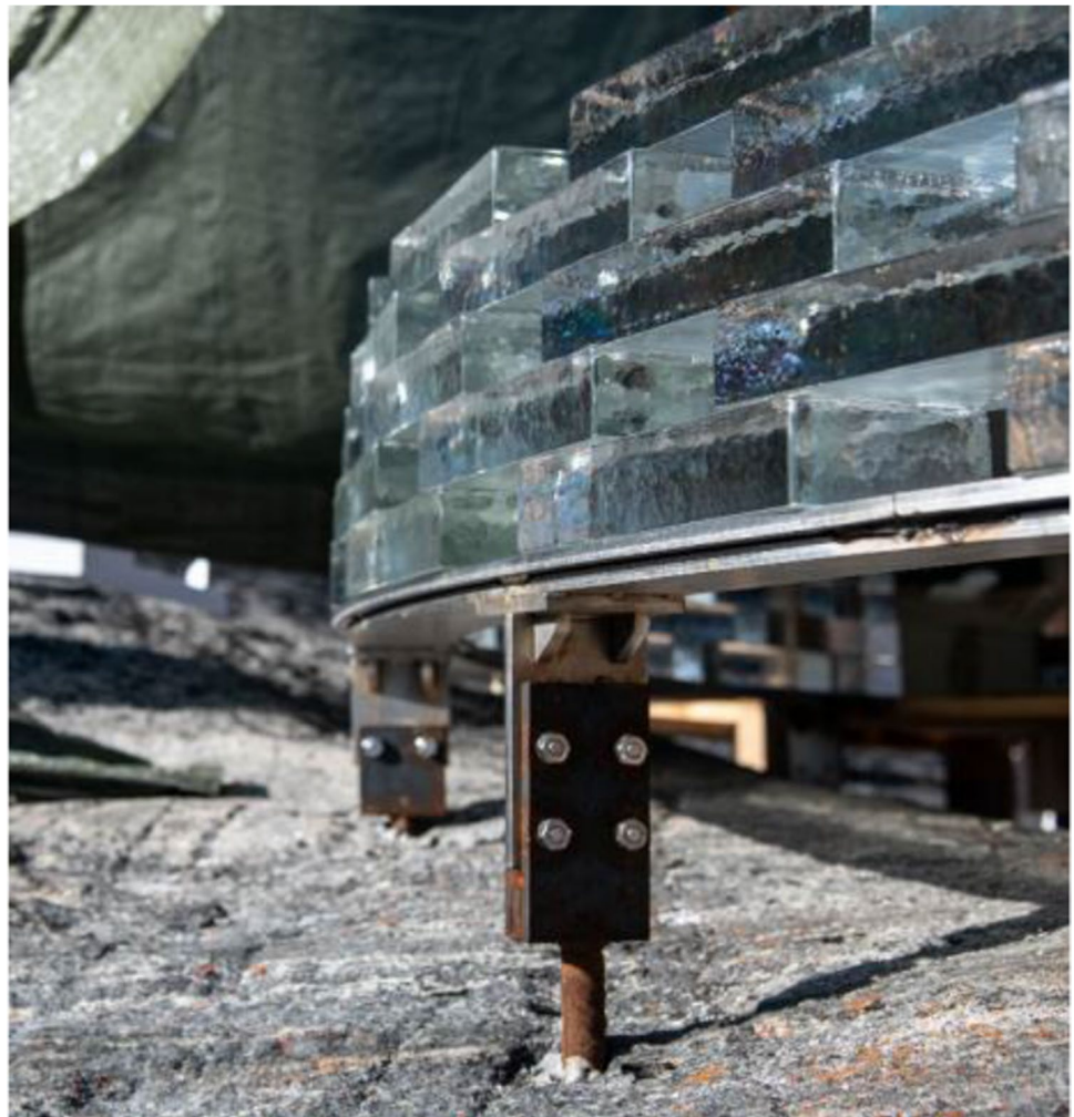
Fig. 22 Foundation of the glass-brick Qaammat Pavillion
