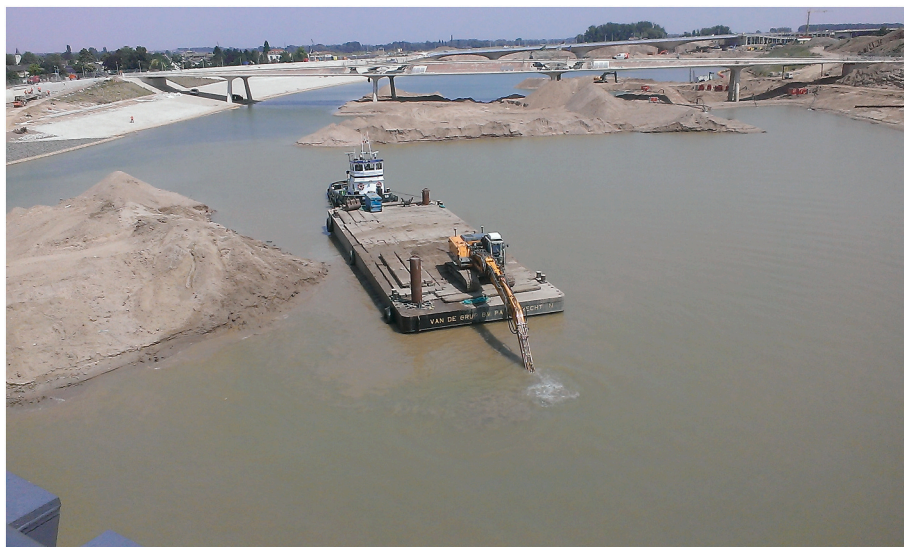
Fig. 7. Excavation of floodway at Nijmegen (July 2015).
