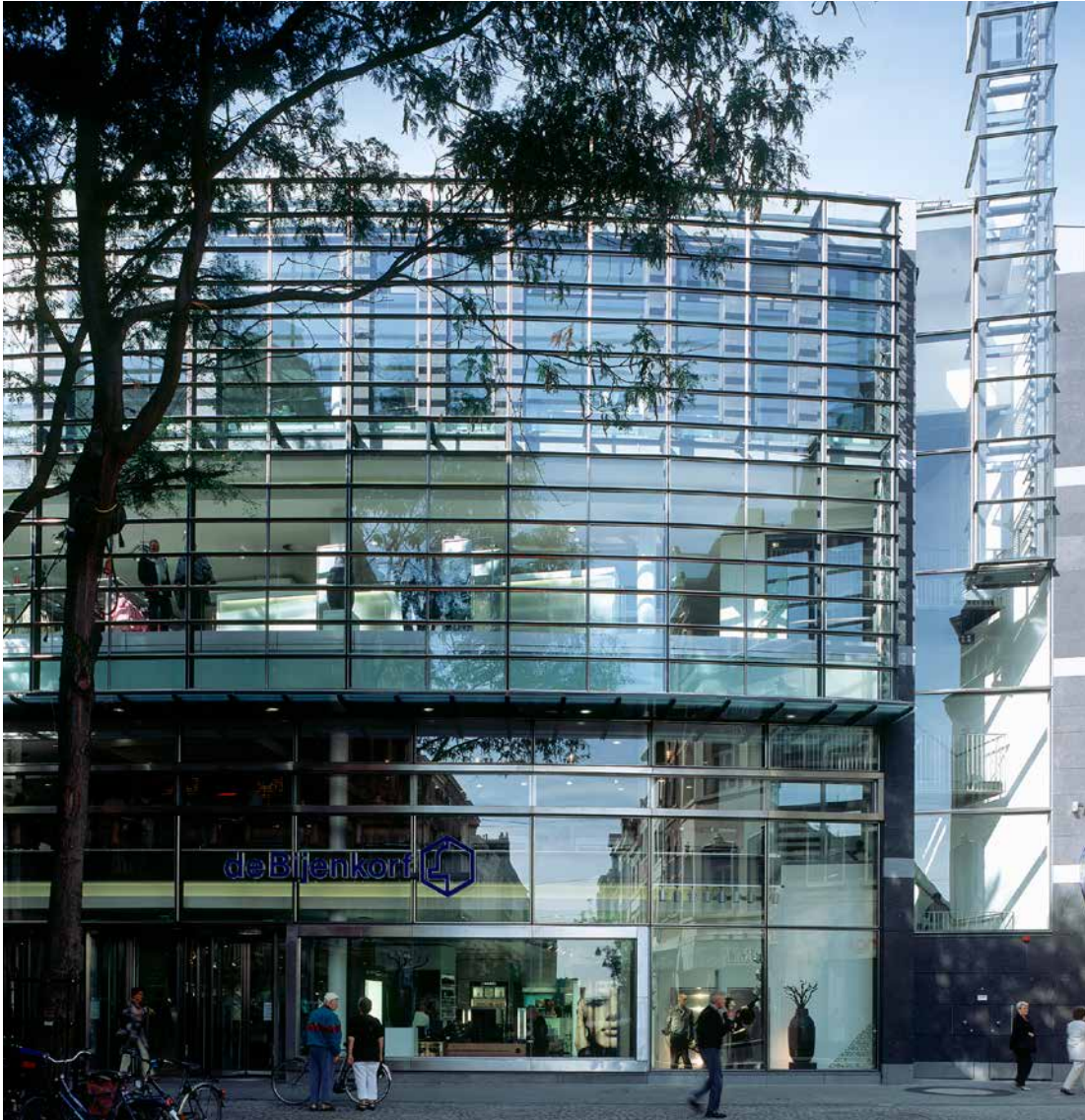
10. PHOTO OF THE CURRENT SITUATION OF THE KERSEMARKT FACADE
