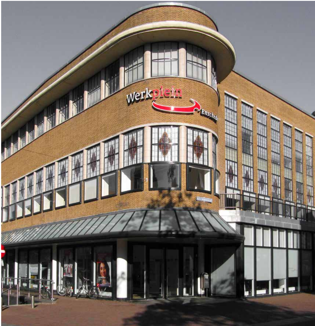
9. PHOTO OF THE CURRENT SITUATION OF THE BRAMMELERSTRAAT FACADE
