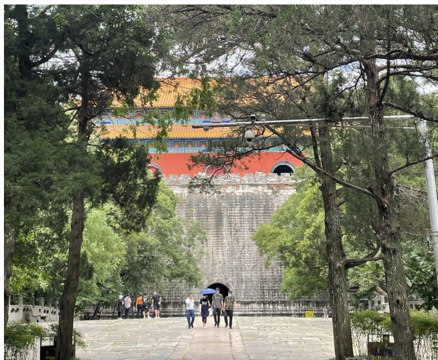
Figure 6. ‘Fang Cheng Ming Lou’ (City Gate Tower) inside The Xiaoling Tomb of the Ming Dynasty. (Source: Authors).
