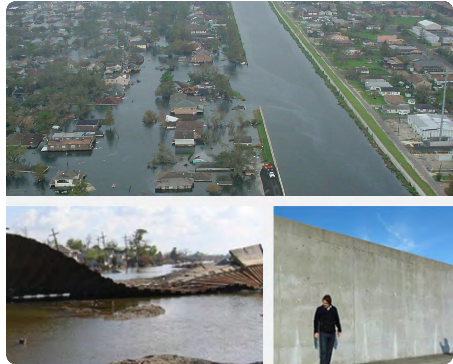
Figure 2: Top and bottom-left: Floodwall failure on 17 th Street Canal from Hurricane Katrina in New Orleans (photos by U.S. Army Corps of Engineers and IPET, 2005 ). Bottom-right: Rebuilt New Orleans floodwall in 2013 (Photo by Bianca Hardeman).
