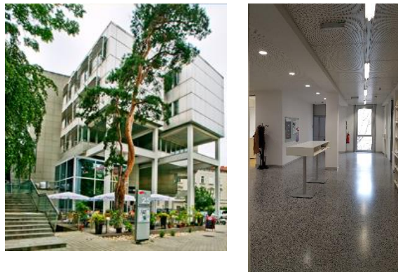
Fig. 3 – TUG- Institute for building physics, services and construction (outside left and inside institute right), Austria
