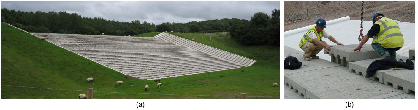
Fig. 1. Prototype stepped spillways with inclined downward steps for Bruton flood storage reservoir, UK ( \theta = 14^\circ , H = 10.75 m, B = 48 m, and Q \approx 250 m 3 /s): (a) general view of the spillway shortly after completion in 2008; and (b) construction details with installation of precast concrete blocks over the geotextile membrane. (Images courtesy of John Ackers.)
