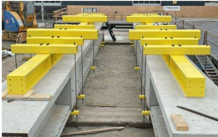
Fig. 6 Specimen with the protection frame
