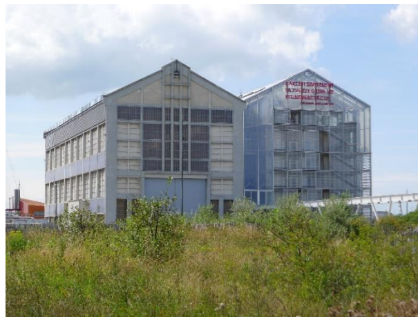
Fig. 3. The FRAC museum in Dunkerque was doubled in space by coping the original hall and leaving it open and creating an optimized museum in the extra volume.
