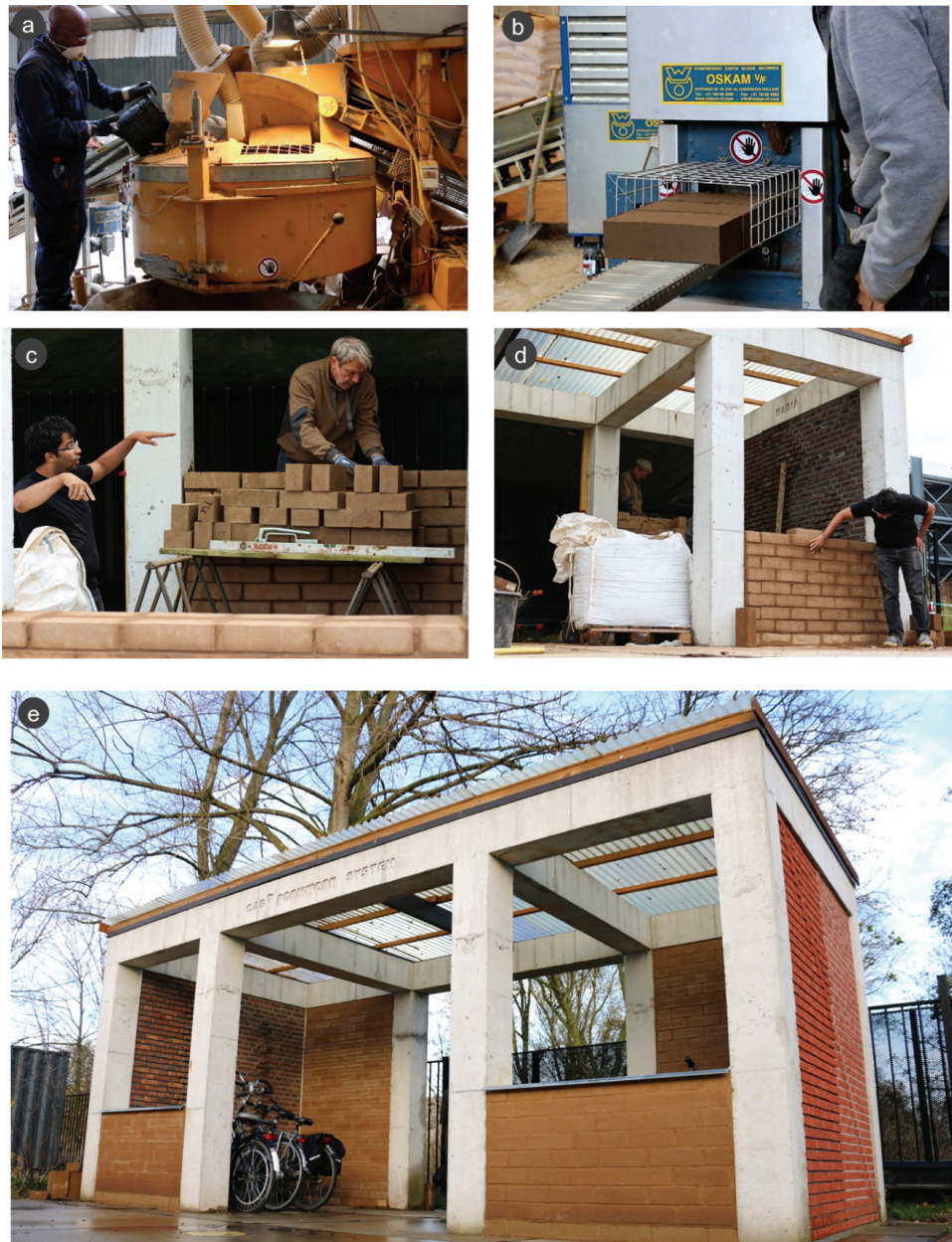
Figure 6.34: Upscaling of CD-CEBs for construction of demonstration walls at the Green village, TU Delft. (a) Mixing of cow-dung and soil, (b) Production of CD-CEBs with a hydraulic press, (c) Masonry with CD-CEBs. The mortar used has the same composition as the CD-CEB but with more water, (d) the fully constructed front wall of CD-CEBs (without the metal roofing) and (e) The finished demonstration structure with an unstabilised wall on left and cow-dung stabilised walls on the right. The demonstration structure is a full-scale test on the performance of the CD-CEB wall as compared to the unstabilised wall. (Image c and d are credited to Justyna Botor).
