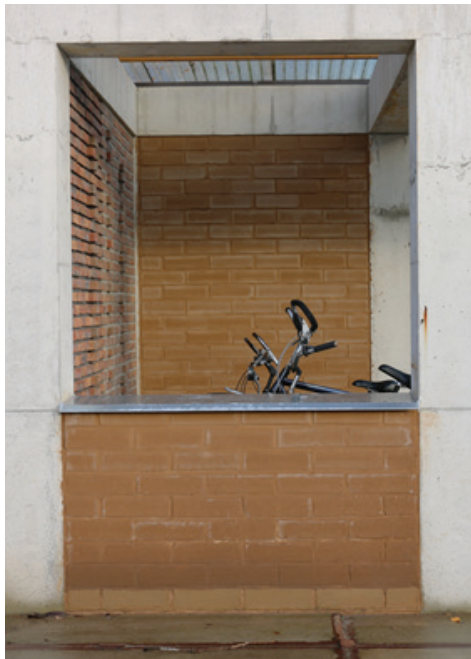
Figure 4.27: Demonstration structure constructed with unstabilised CEB at The Green Village, TU Delft. The wall in front is exposed to rain whereas, the wall behind is protected with a roof. The bottommost layer of both walls is composed of lime stabilised earthen blocks to prevent direct contact with the concrete slab (and pooling water in the vicinity of the wall). It can be observed that the bottom region of the front wall is much wetter (via the darker colour), probably due to splashbacks or capillary rise (although a damp coat was applied over bottom-most blocks).
