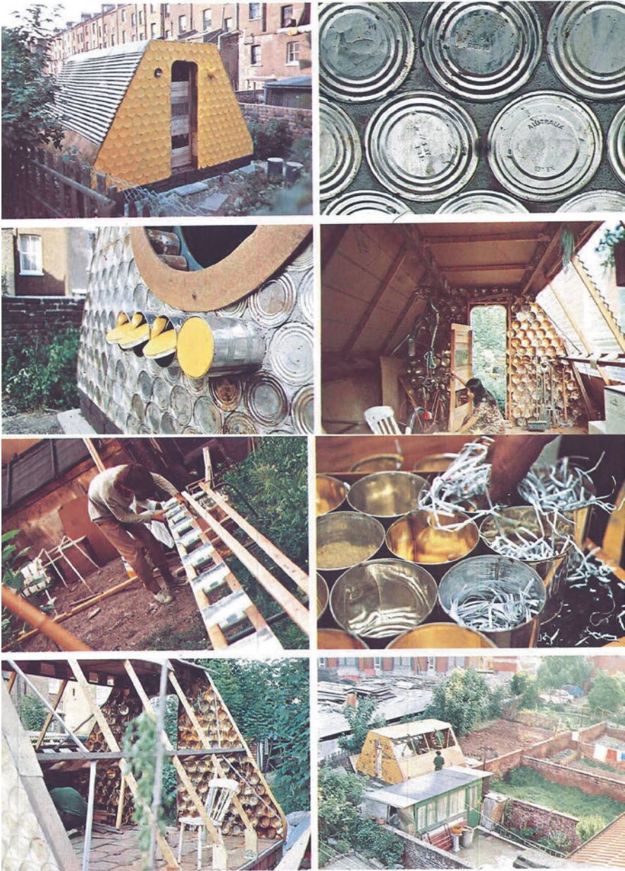
Fig. 10.1 Small house in London, SUG, details from the inside and the outside of the reused tin-can wall, tin-can structural beam, reused tin cans filled with shredded paper, and location of the house in the backyard. (Source: Kan and Poteliakhoff 1975)
