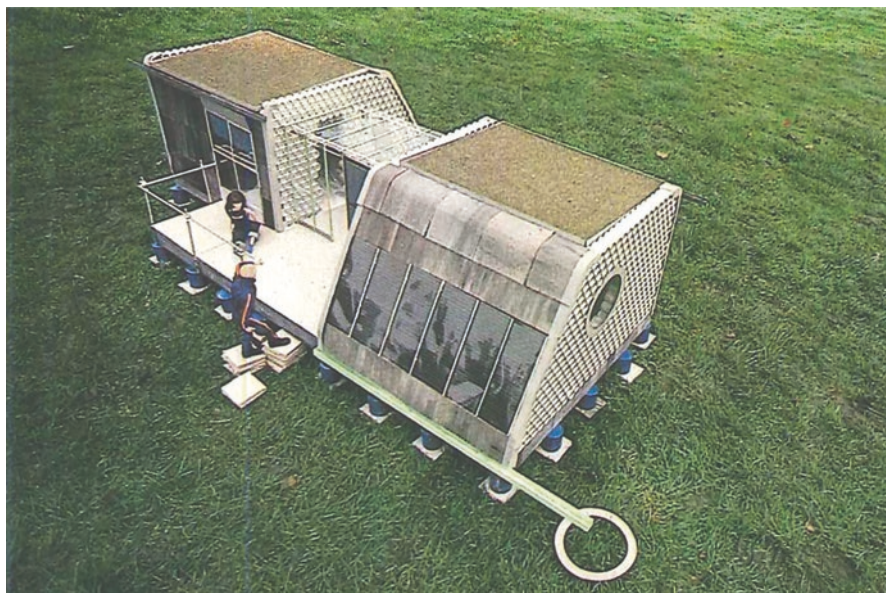
Fig. 10.5 Two-person dwelling, SUG , south-east side, pending wall with solar collectors. (Source: Kan 1978)
