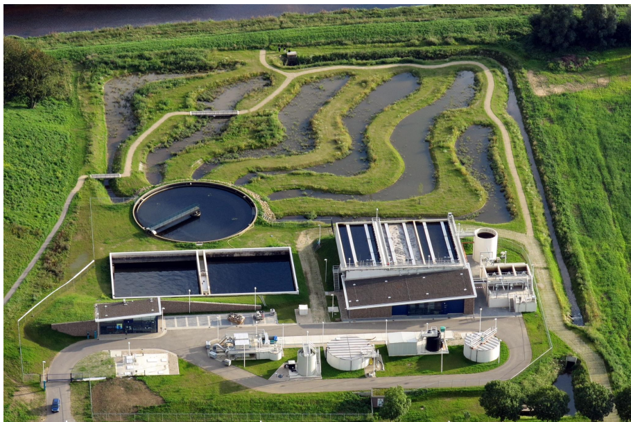
Figure 4.2: Photograph of the wastewater treatment plant in Dinxperlo. The Nereda ® reactors are located on the right, attached to the building with the sloped roof. The sludge buffer and the sand filter are located to the right of the Nereda ® reactors. The inlet works, including the influent buffer are located at the bottom. The old pre-existing aeration tank and clarifier on the left are now part of a public water garden (on the top).
