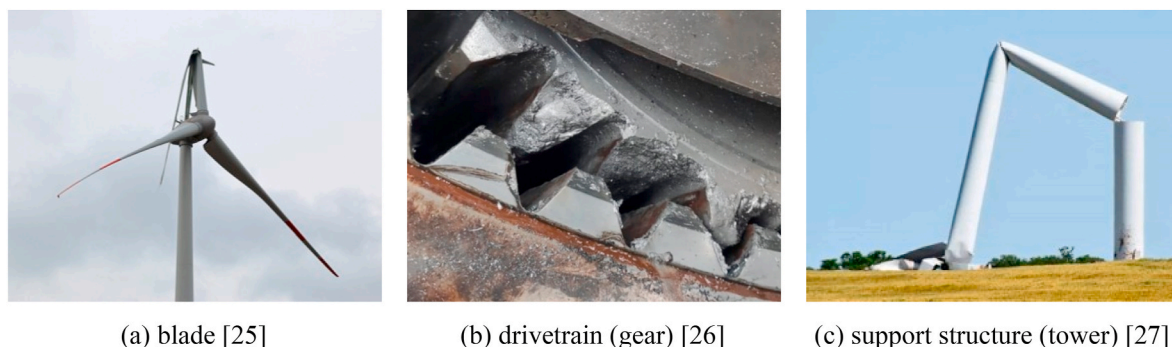
Fig. 4. Typical wind turbine fatigue failure cases [25–27].
