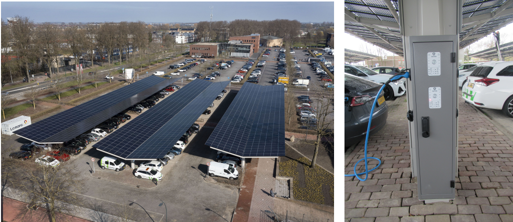
(a) PV array at the solar parking lot located at the municipality building of Dronten, the Netherlands (b) Charging station with 4 charge points
