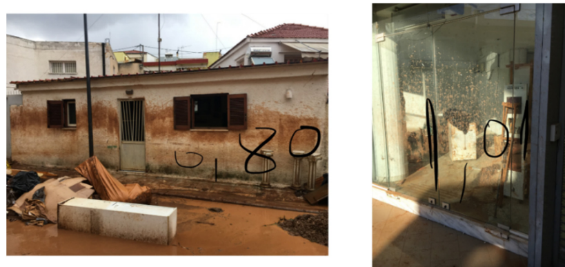
Figure 6. Uncertainty issues at the observation points: the finally selected values for the observed maximum depths are 0.80 m (left), 1.01 m (right).
