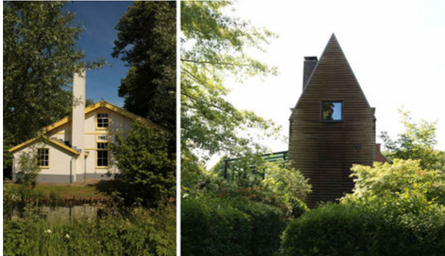
FIG. 4.87 Utrecht (NL), Fort Blaukapel: reuse of historic buildings (left) and new constructions (right) (F. Marulo 2019)
