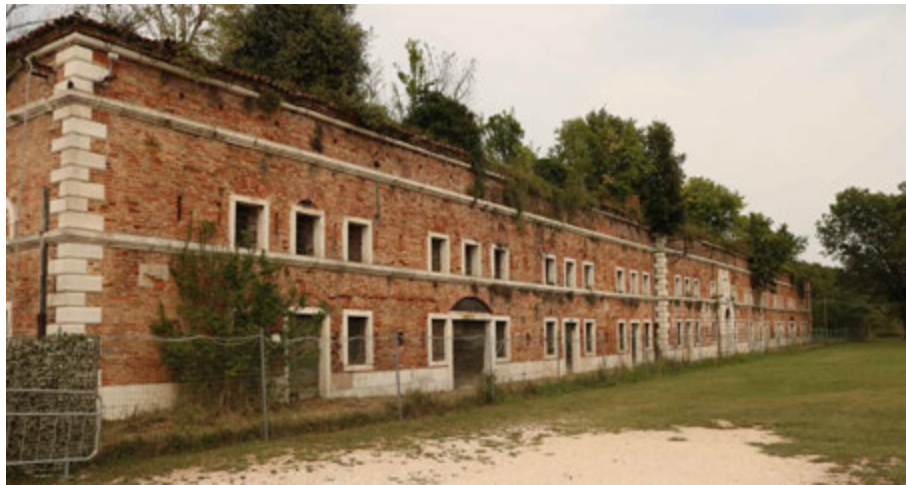
FIG. 5.51 Venice (IT), Forte Marghera: French barracks (8), southern façade (F. Marulo, 2020)
