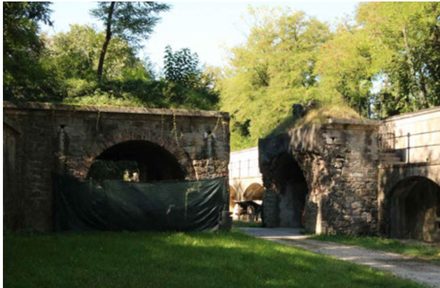
FIG. 5.15 Venice (IT), Forte Gazzera: one of the arches formerly connecting the central crosspiece to the perimeter structures and partially demolished during the German occupation (1943-1944) (F. Marulo 2020)
