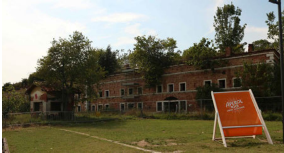
FIG. 5.50 Venice (IT), Forte Marghera: French barracks (9), southern façade (F. Marulo, 2020)
