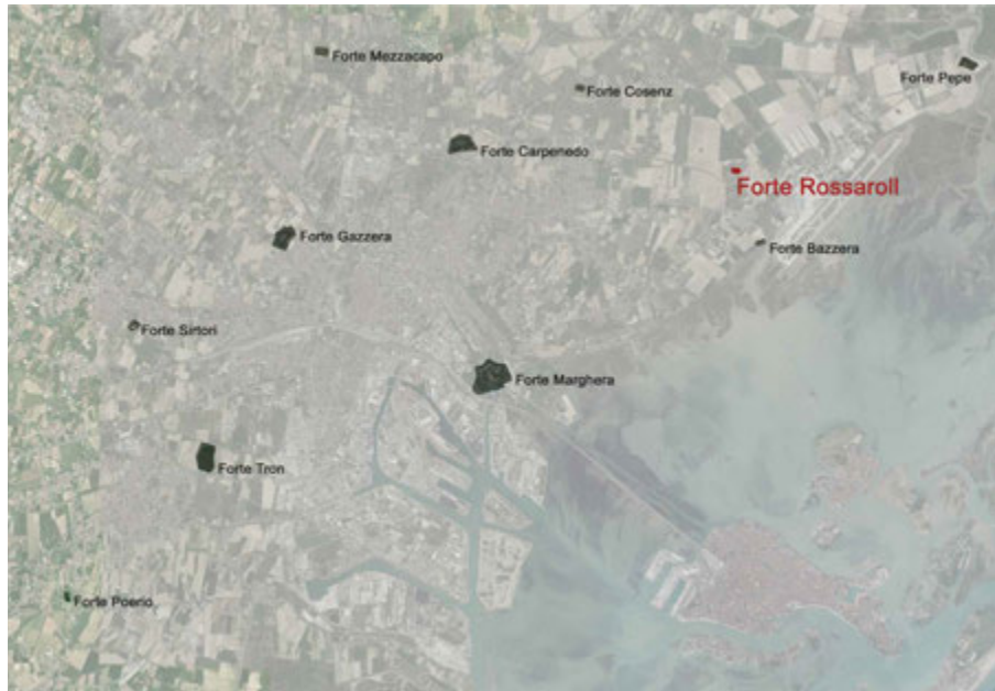
FIG. 5.83 Venice (IT), Forte Rossaroll: location in the Entrenched Field of Mestre (aerial image retrieved at: https://geoportale.comune.di.venezia.it [05.06.2020]) (F. Marulo 2020)
