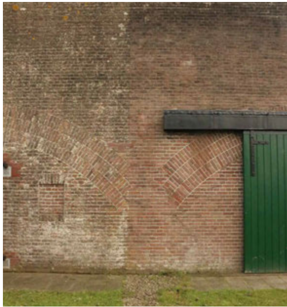
FIG. 4.50 Bunnik (NL), Fort bij Vechten. Bombproof barracks: partial cleaning of the façade in the portion falling within the strook (strip) (F. Marulo 2020)
