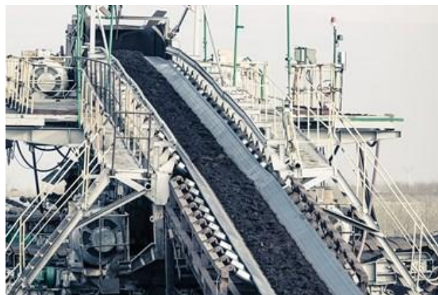
Figure 1.1 Transferring of iron ore from a belt conveyor through a transfer chute [2]
