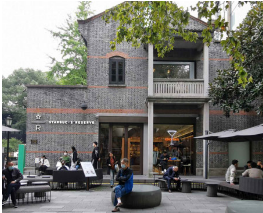
FIG. 6.28 The symbolic Starbucks since the completion of Xintiandi, and has been a prominent landmark in this district. Source: author, 2021.
