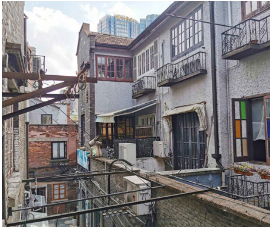
FIG. 7.23 A view of the second and third layers of the lilong houses. Source: author, 2021.
