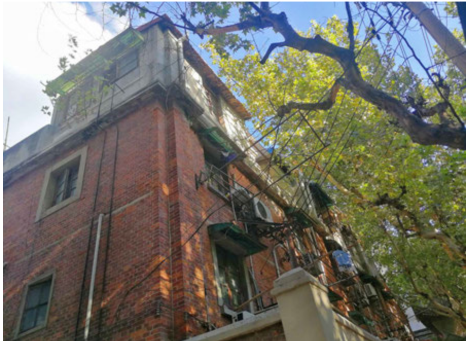
FIG. 8.26 The additional one floor on the top of the original building with grey in colour and plaster in material, replacing the red bricks. Source: author, 2018.
