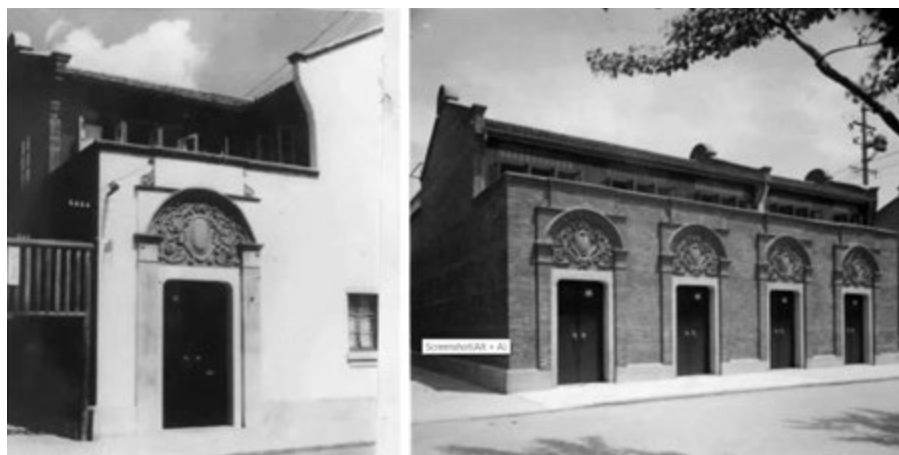
FIG. 6.10 [Left] The site of the first national congress of the Chinese Communist Party after the first simple repair in 1952. [Right] The site after restoration and conservation to its 1921 appearance in 1958. According to memories of Li Shucheng’s wife Xue Wenshu (薛文淑), and Dong Biwu, delegate to the First Congress, the façade along Xingye Road and decorations of the four shikumen pediments were restored to the original looks. Source: Centre for the Protection of Historic Buildings in Shanghai, available at https://www.sohu.com/a/474942957_260616 , accessed on 10 August 2021.
