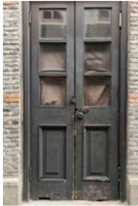
FIG. 6.13 Conserved gate plank and changed new hardware door connecting shaft. Source: author, 2021.
