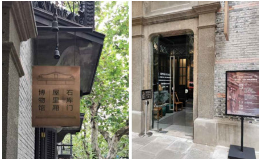
FIG. 6.19 The front façade elements of the Open House Museum to present scenes from the life in shikumen wulixiang. From the balcony (left) and the gate frame (right), the features of the historical shikumen housing can be perceived by visitors. Source: author, 2021.
