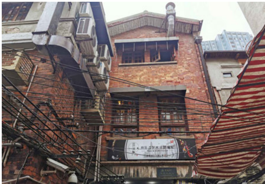
FIG. 7.27 The one-storey high wire network, antipathetic iron-sheet exhaust chimneys, and air conditioning units stacked one on top of the other in Tianzifang. Source: author, 2019.
