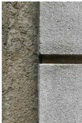
FIG. 6.15 Conserved gate frame made of original architectural materials. Source: author, 2021.
