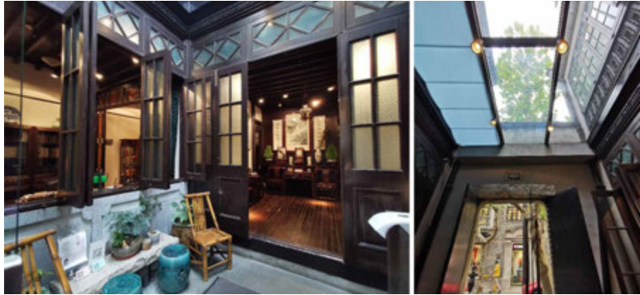
FIG. 6.23 The entrance courtyard and the added glass top cover. Source: author, 2021.
