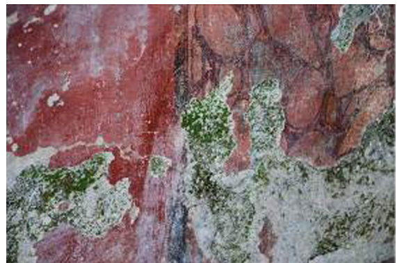
Fig. 8 Detachment and loss of a lime-based plaster from the masonry support. Archaeological site of Dion, Greece (Roman period): Plaster consisted of two layers of a total thickness of 2.5 cm (external: 0.5 cm, internal: 2 cm), decorated with wall paintings. (Photo archive: Lab. of Building Materials AUTH)
