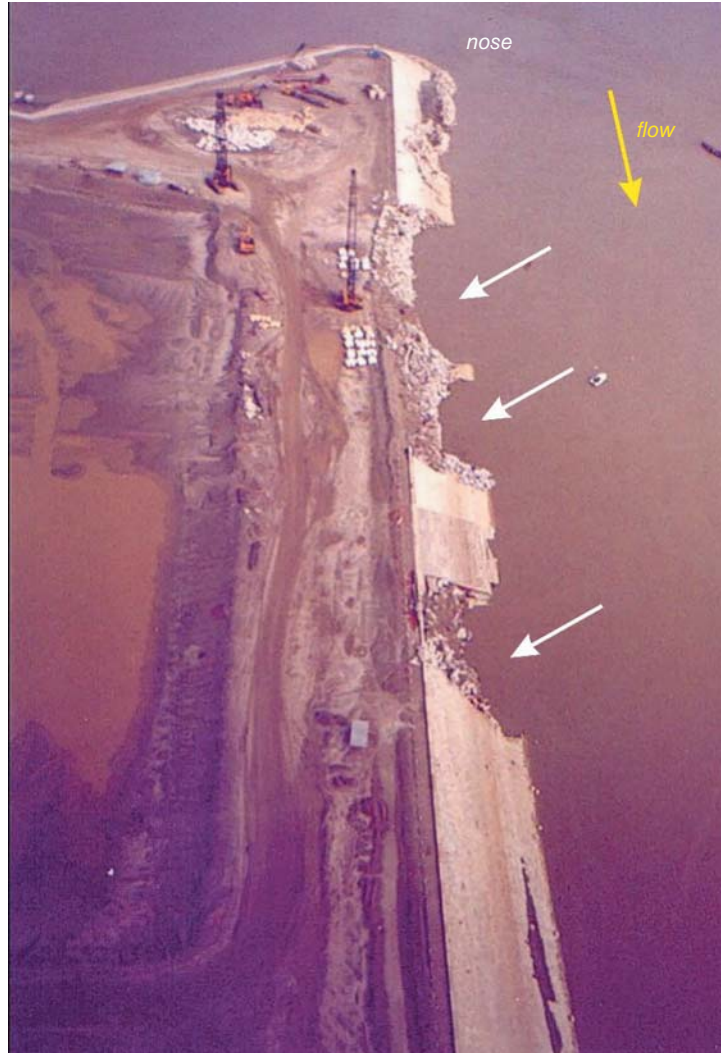
Figure 20.34 Image of the B2 hardpoint in 1998 showing the multiple failures (white arrows) formed at the height of the 1998 flood. Flow towards viewer and the upstream nose of the B2 hardpoint is labelled. Source: Photograph courtesy of Mr. Bob Courtier, W.S. Atkins Ltd.
