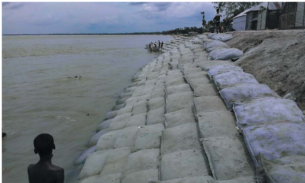
Figure 20.35 Sand-filled geotextile bags, or geobags, used for bank protection at Chauhali, Jamuna River. View looking upstream.
