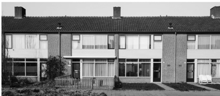
Figure 1. Typical Dutch Unreinforced Masonry (URM) terraced houses [ http://www.bestaandewijk.nl/tag/jaren-60-wijk/ - Roel Simons (photographer)].
