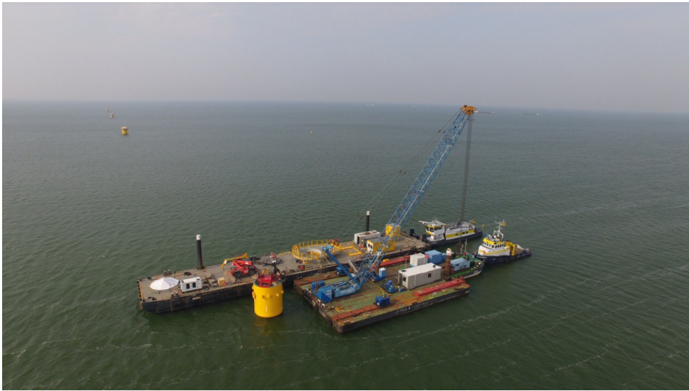
Figure I.6: Aerial photo of the shaker on the monopile (MP45) tested as part of the DISSTINCT project in the Westermeerwind wind farm. Source: Versteijlen et al., 2016a
