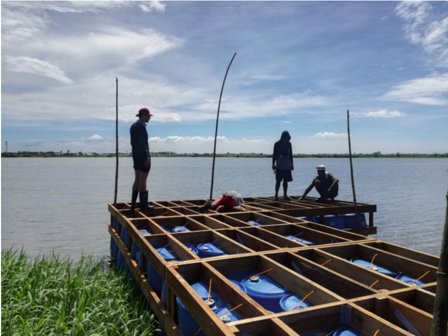
Fig. 6 Floating foundation modules
