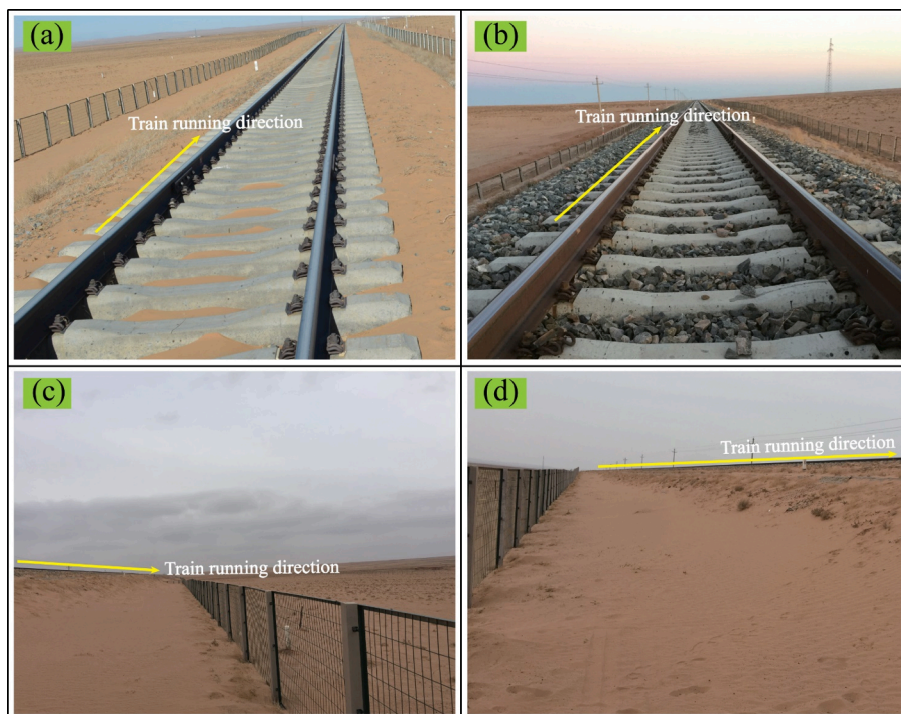
Fig. 2. Site conditions: (a) sandy section, (b) clean section, (c) Front view of train operation direction, (d) Back view of train operation direction.
