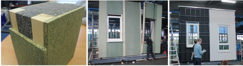
Figure 10.5 (A) sample of the prefabricated sandwich panel. (B) Left and right panel attached to the substructure, through timber sticks. (C) Testing different cladding material.
