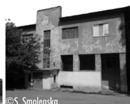
HOUSES FOR EMPLOYEES
