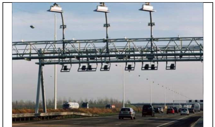
Fig. 1. License plate detection of Camera detection of a road pricing system
