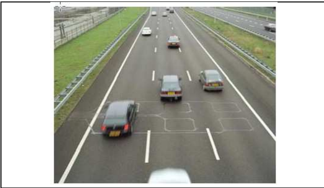
Fig. 12. Highways in the Netherlands with electrical wires in the surface of the road to assess traffic density
