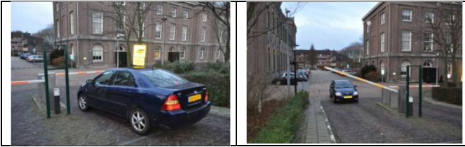
Fig. 11. Entrance barrier at the Netherlands Defence academy at Den Helder
