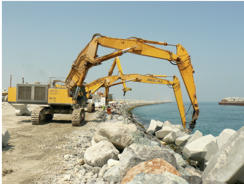
Figure 13-24 Construction workfront with several cranes, requiring access by dumpers (Van Oord)
