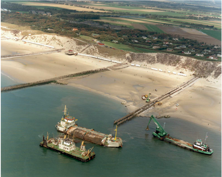
Construction of a beach groyne (courtesy Boskalis)
