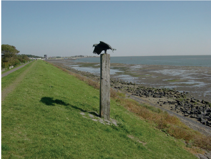
Figure 11-26 Dike with grass revetment (Vlieland, photo Waterboard Fryslân)
