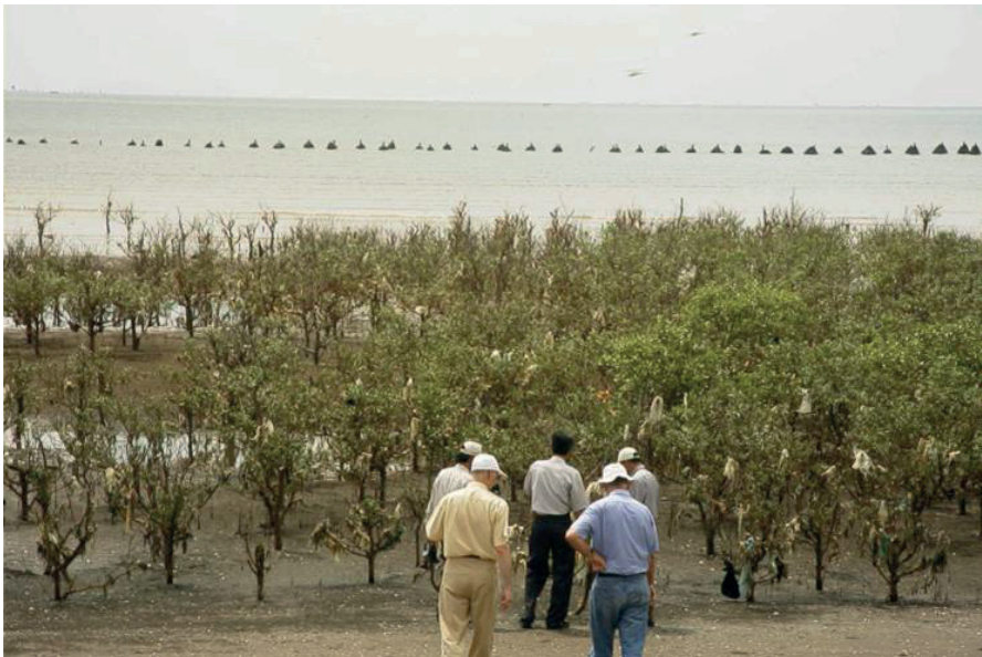
Figure 12-20 Mangrove reforestation with wave load reductor
