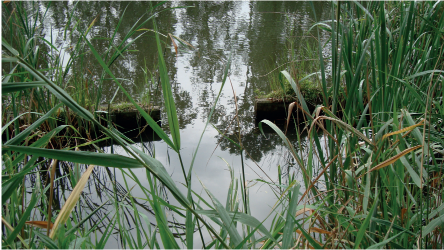
Figure 12-5 Gap in a sheetpile, in this case especially to allow beavers to cross the sheetpile (photo Verhagen)
