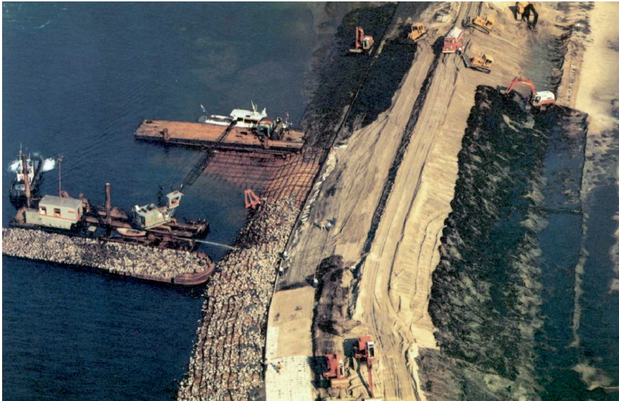
Figure 13-16 Placing fascine mattress on revetment
