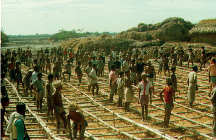
Figure 13-9 Construction of bamboo mattress
