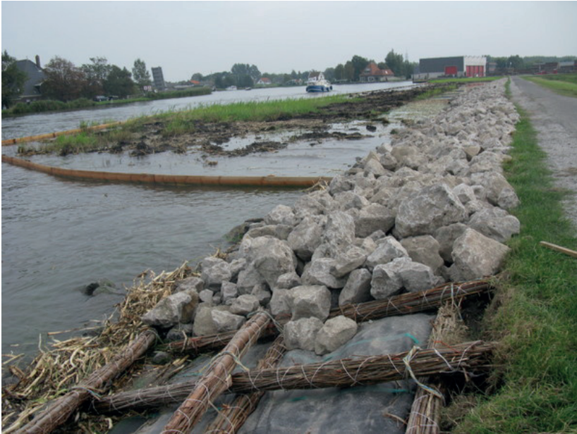
Figure 11-8 Geotextile under mattress (photo Griendhouhandel)
