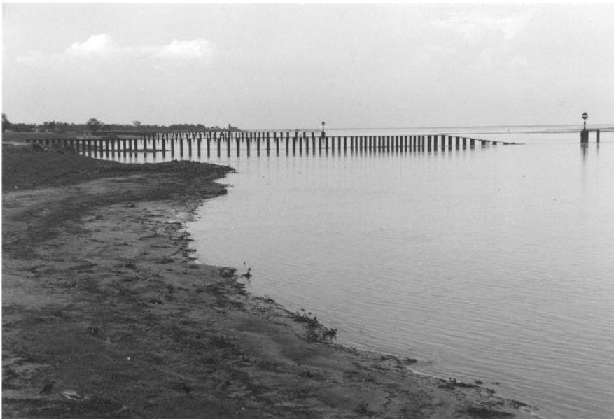
Figure 11-22 Pile screens in Jamuna river Bangladesh (Photo Van der Wal, 2000)
