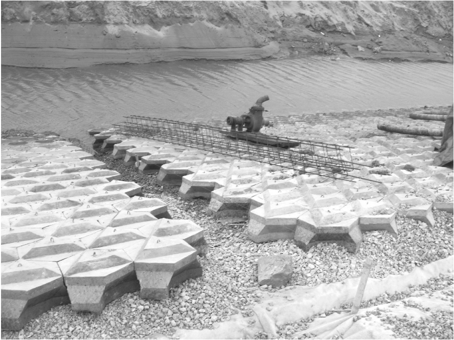
Figure 8-22 Interlock blocks applied in Vietnam (photo Verhagen)
