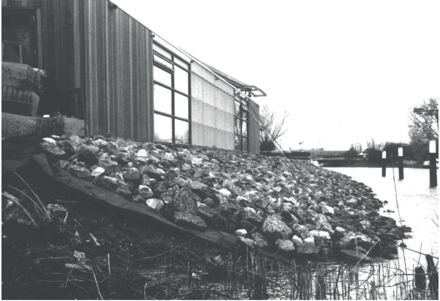
Figure 11-16 Simple bank protection with geotextile
