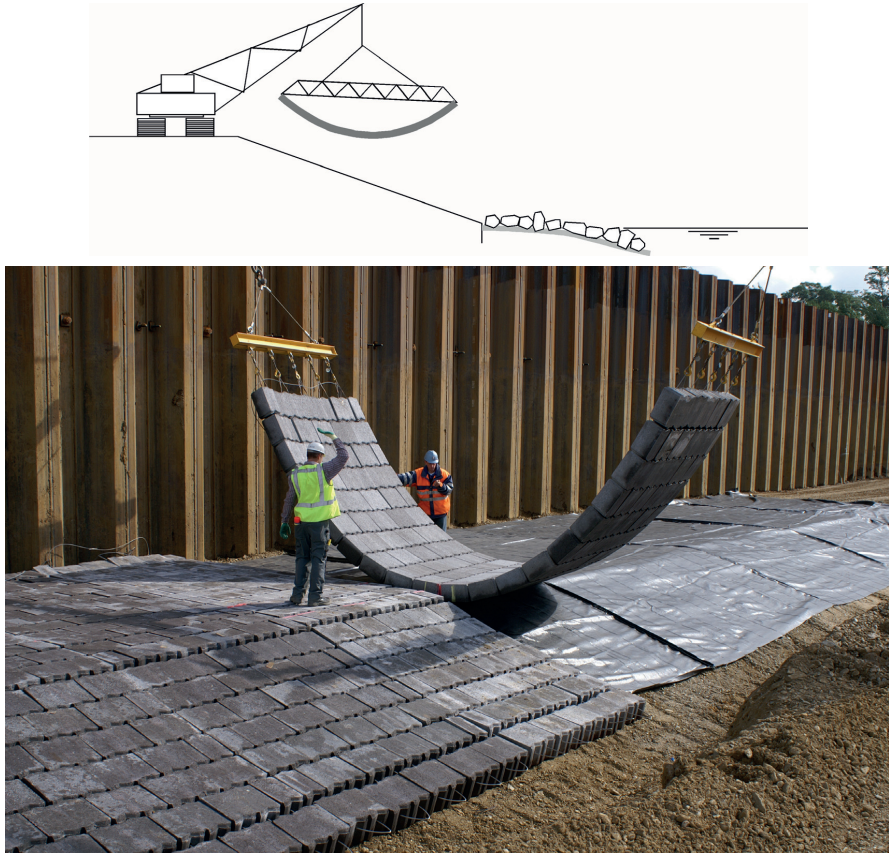
Figure 13-18 Placing of prefabricated mat on revetment (Dycel blockmat)
