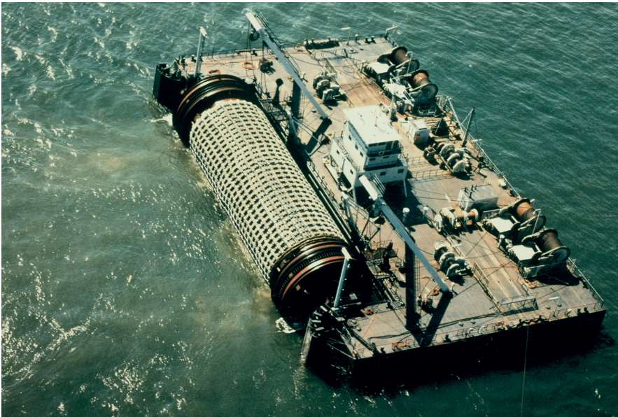
Figure 13-10 Sinking block mat in Eastern Scheldt (Rijkswaterstaat)
