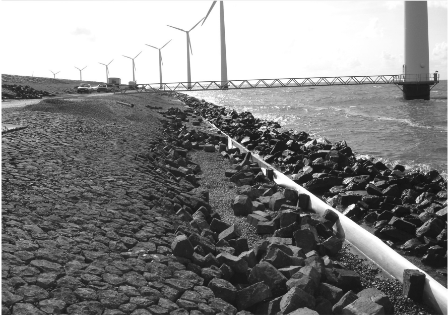
Revetment improvement works near Lelystad (photo W. de Vries)
