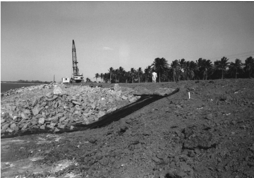
Figure 11-23 Loose rock dike revetment (Nickerie, Surinam, photo L. Philipse)
