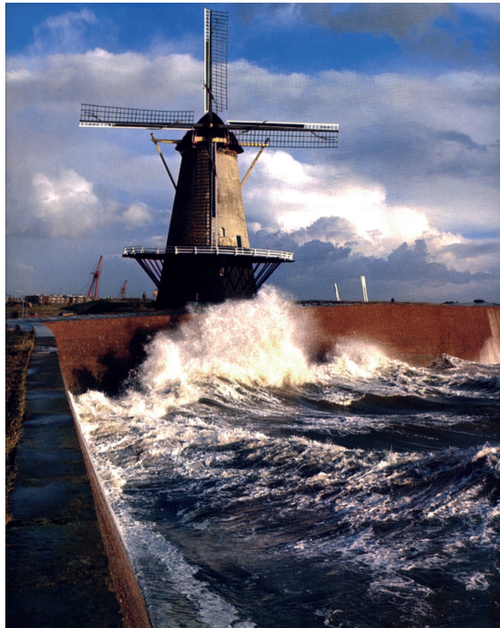
Figure 11-27 Seawall (Vlissingen, photo Wil Riemers)
