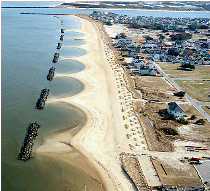
Figure 11-32 Offshore breakwaters (East Beach, Norfolk, Virginia; photo SirFin, Panoramio)
