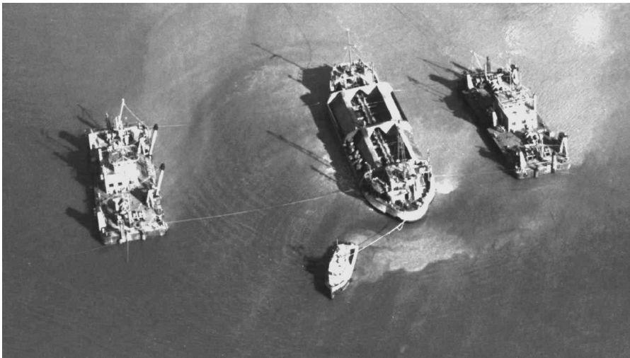
Figure 13-8 Sinking fascine mattress
