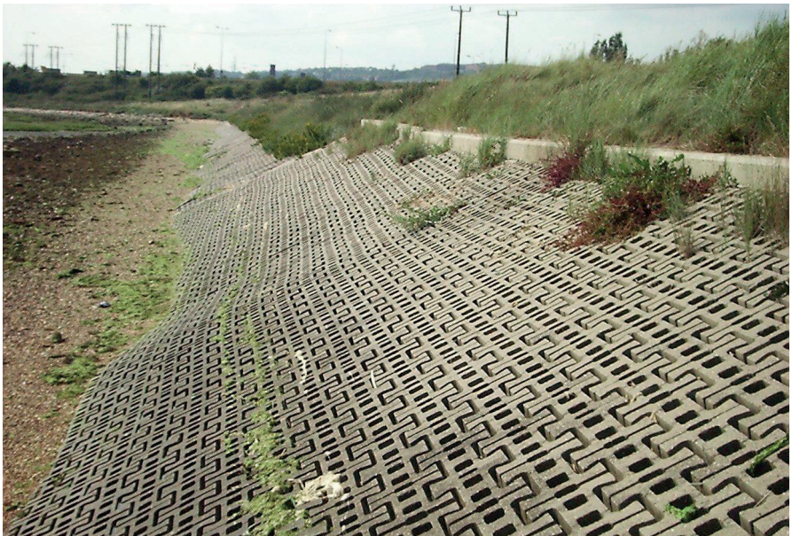
Figure 11-17 Block mat as bank protection (photo Armortek UK)
