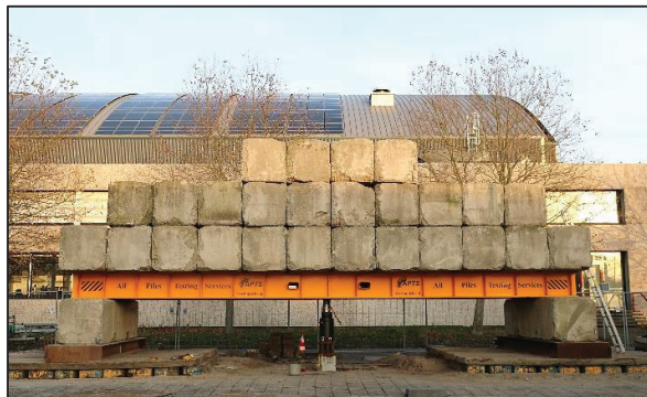
Figure 6. Deadweight test frame system used at the Delft test site
