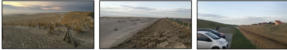
Fig. 2 Photo sequence of coastal flood defenses near Petten, the Netherlands. From left to right: seaward side of the Hondsbossche Dunes (left), back-dune fronting the dike (center), and backside of the dike (right). (Photos by J. Figlus.)
