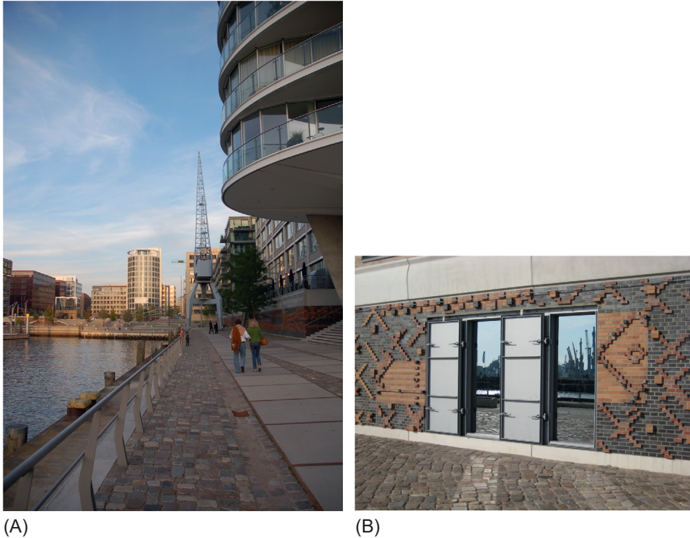
Fig. 2 Modern version of mount settlements: flood proof development Hamburg HafenCity along the river Elbe. (A) Building with elevated ground floor, Hamburg HafenCity, Sandtorhafen. (B) Hamburg HafenCity, Flood-proof doors at ground level. ((A) Photo by Defacto Urbanism, Rotterdam. (B) Photo by Defacto Urbanism, Rotterdam.)
