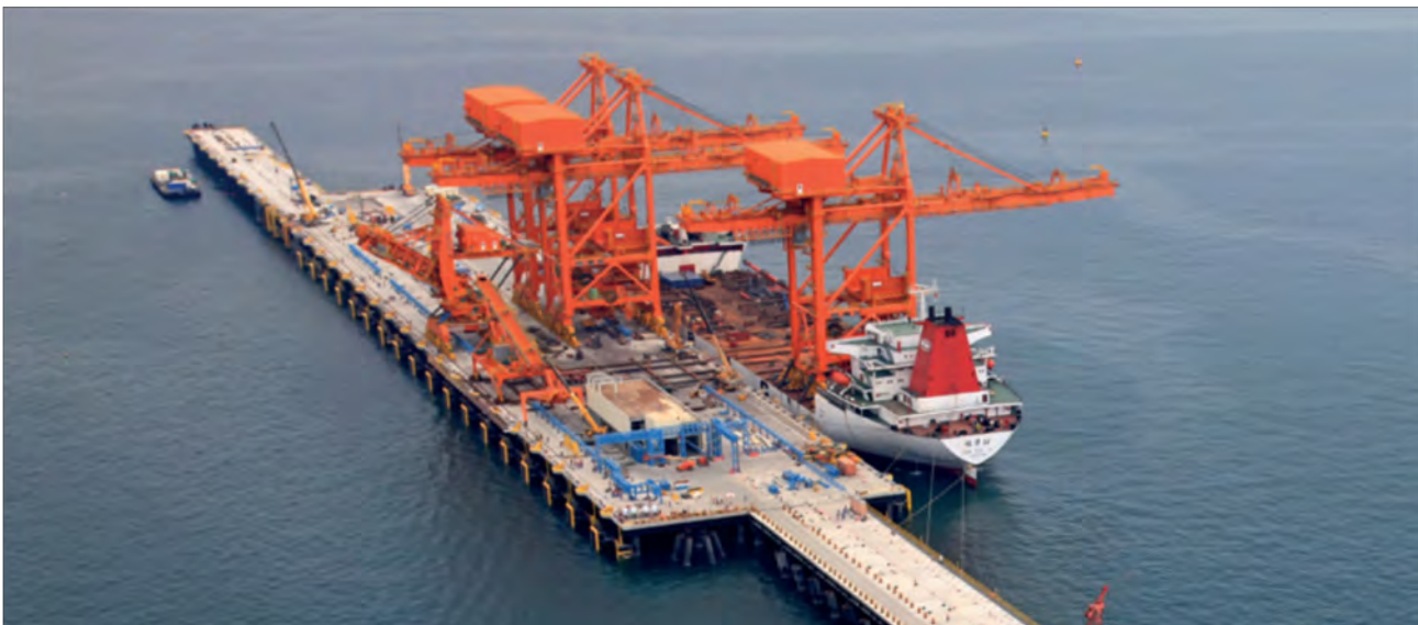
Figure 5.20: Iron ore terminal, Port of Sohar, Oman ( Bulk IJzerertsterminal in de haven van Sohar (Oman) by Royal HaskoningDHV is licenced under CC BY-NC-SA 4.0).
