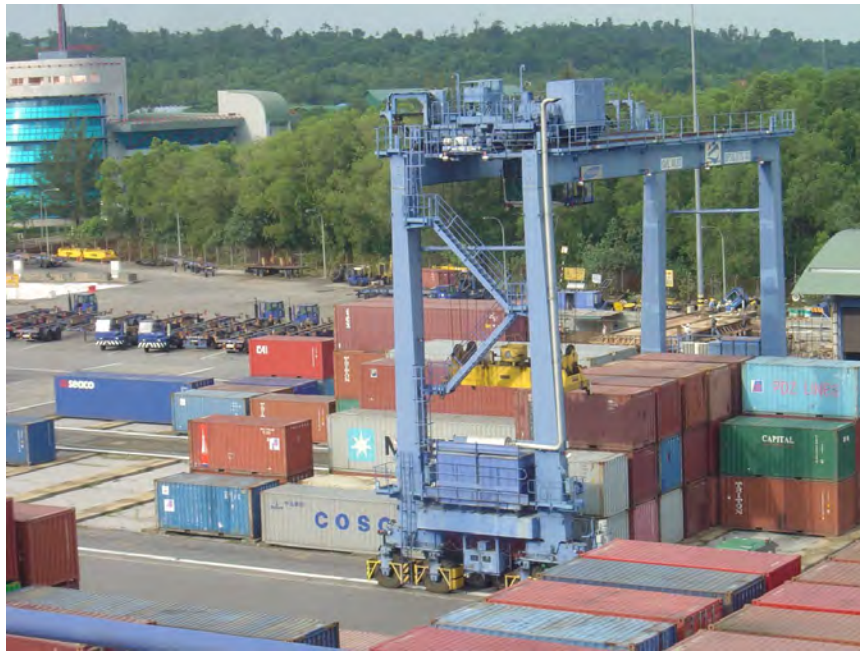
Figure 4.22: Rubber Tired Gantry crane (RTG) (RTG at Bintulu International Container Terminal (BICT) by R.W. Sinyem is licenced under CC BY 2.0).
