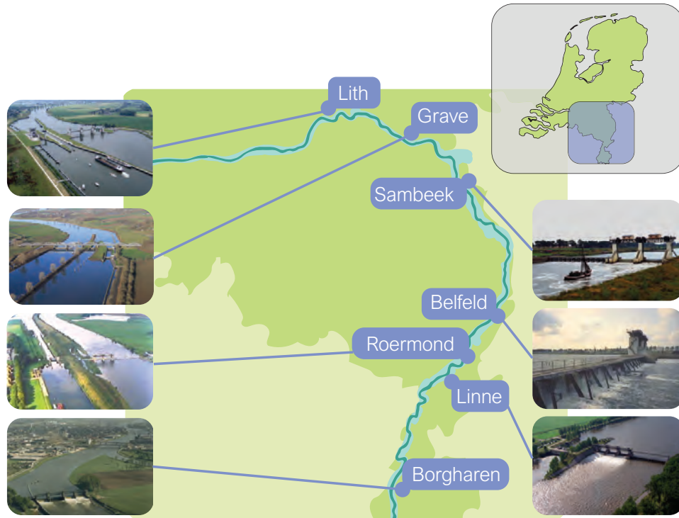
Figure 2.38: Canalised river Maas, the Netherlands (by TU Delft – Ports and Waterways is licenced under CC BY-NC-SA 4.0).
