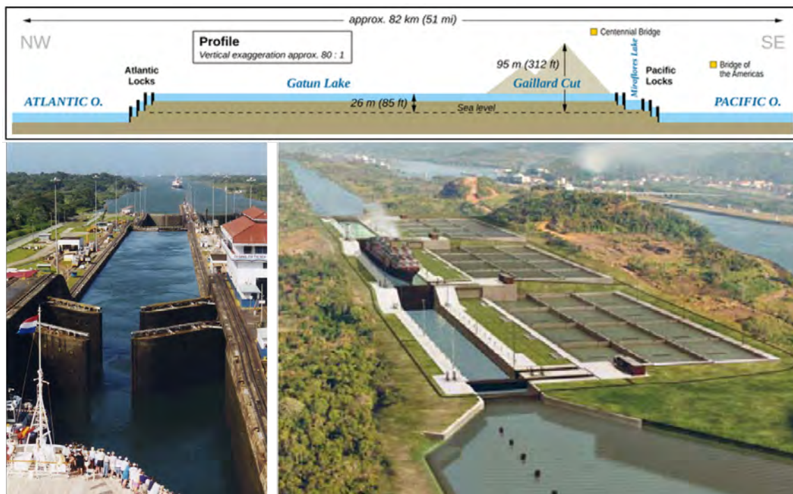
Figure 1.5: The Panama Canal. Top: longitudinal profile; bottom left: the oldest Gatún locks (Atlantic lock system); bottom right: the newest Cocoli locks (Pacific lock system) (source top panel: Panama Canal Map EN by Thomas Rmer is licenced under CC BY-SA 2.0; source bottom panels: Panama Canal Gatun Locks opening by Stan Shebs is licenced under CC BY-SA 3.0 and ACP conceptual view of the Third Set of Locks 02 by Autoridad del Canal de Panama is licenced under CC0 1.0).
