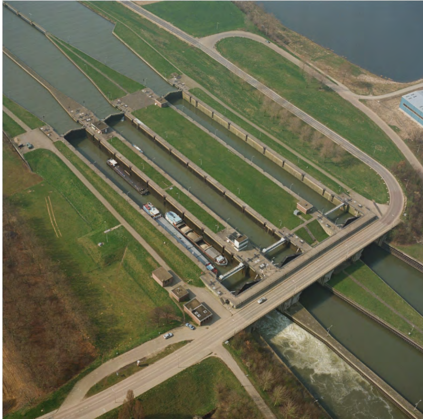
Figure 3.2: Locks at Lith for commercial traffic at the Maas river ( image by https://beeldbank.rws.nl , Rijkswaterstaat, by: Bart van Eyck).
