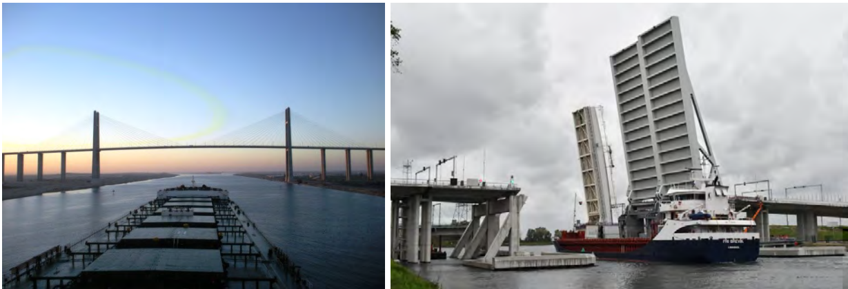
Figure 1.25: Left: Fixed bridge across the Suez Canal (by Aashay Baindur is licenced under CC BY-SA 3.0); right: Movable bascule bridge (by Tvx1 is licenced under CC BY-SA 4.0).
