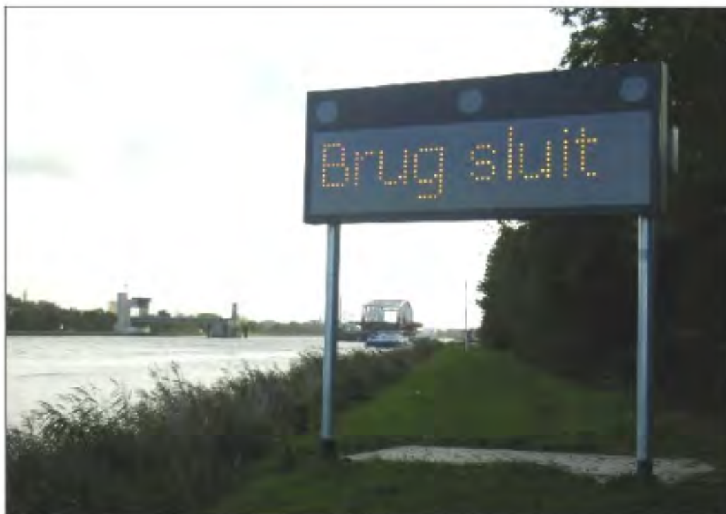
Figure 5.6: Example of a DRIP, saying: ‘Bridge closes’ (image from Rijkswaterstaat ).
