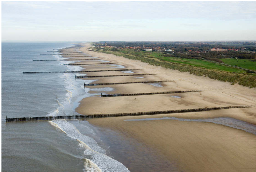
Figure 10.13: Groynes on the Dutch southwestern delta coast, near Domburg, in November 2005. Photo from Rijkswaterstaat ( Credits on page 575).
