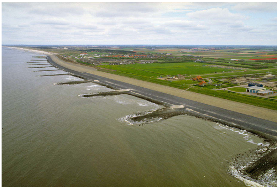
Figure 10.29: Hondsbossche and Pettemer sea defence, The Netherlands, in June 1993. From Rijkswaterstaat ('Credits' on page 575).
