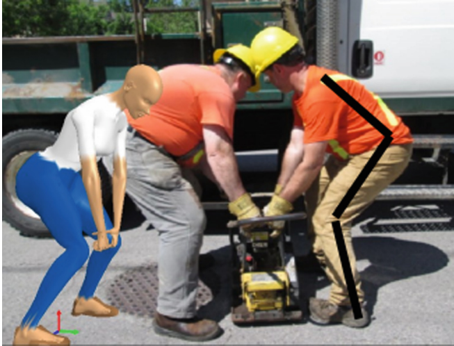
Fig. 3. A photo showing two outdoor workers “maintaining the low back curve” while lifting a plate tamper
