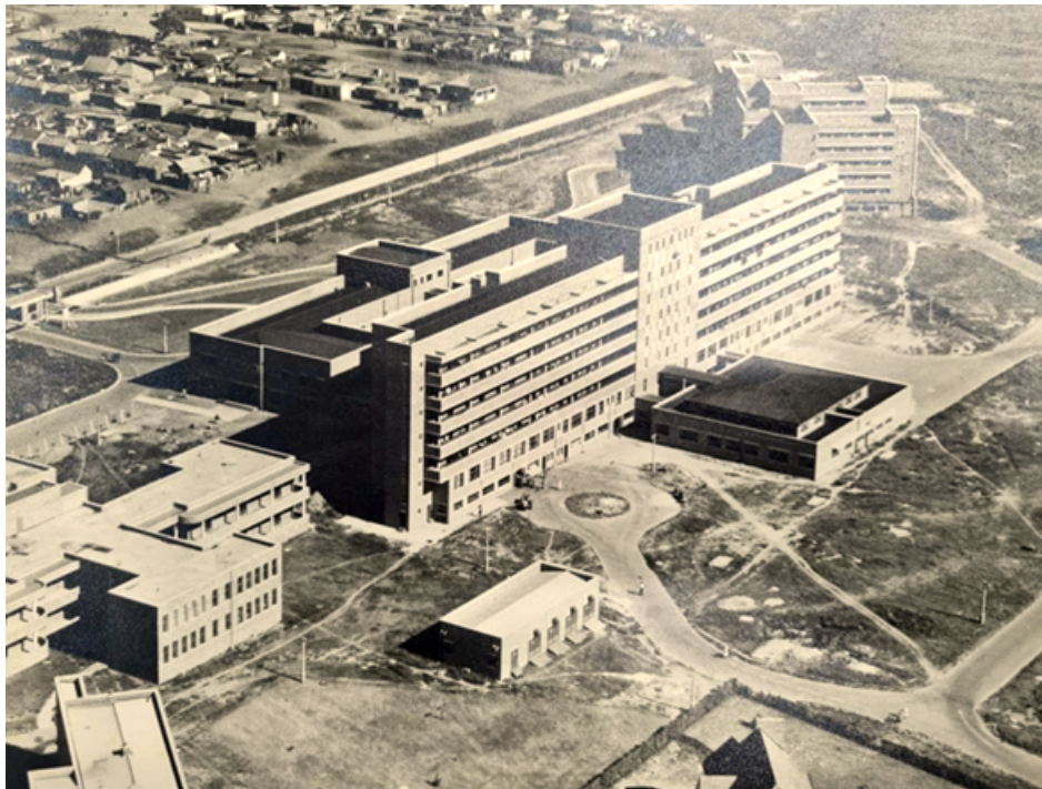
Figure 8. The main ward of the Livingstone Hospital, East London (Source: B. Brinkman, with permission)
