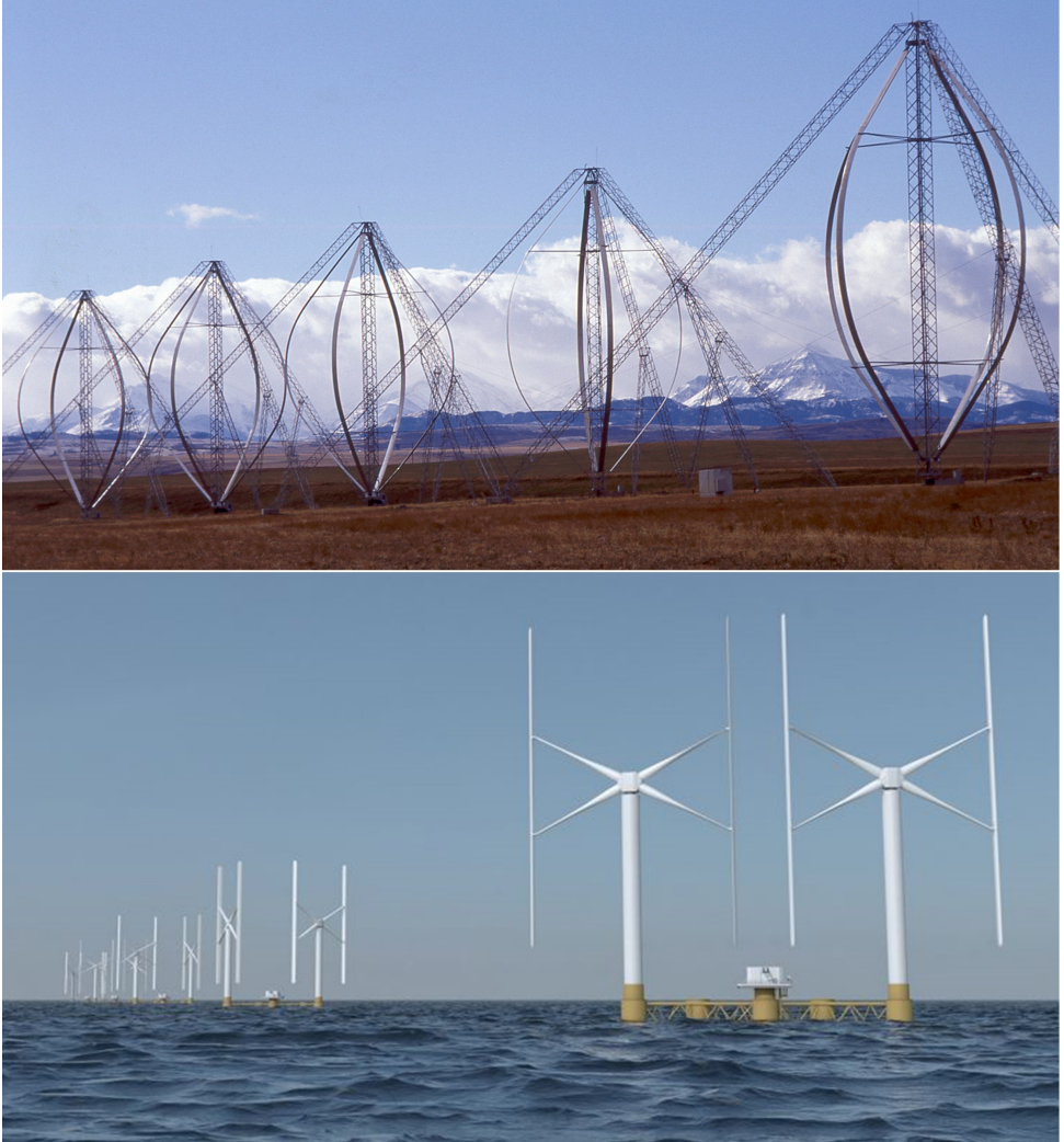
Figure 1.2: Upper: Adecon AL-38 turbines in Pincher Creek, Alberta. Photo by Jos Beurskens (Möllerström et al., 2019). Lower: The NENUPHAR concept of floating VAWT with a double 2 \times 5 MW rotor concept.
