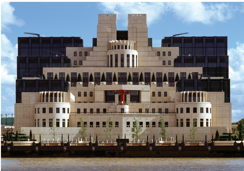
Figure 10. Photograph of the SIS Building in London, seen from the River Thames, and taken on 1 January 1994, shortly after the building's completion. © Bildarchiv Monheim GmbH/Alamy Stock Photo.
