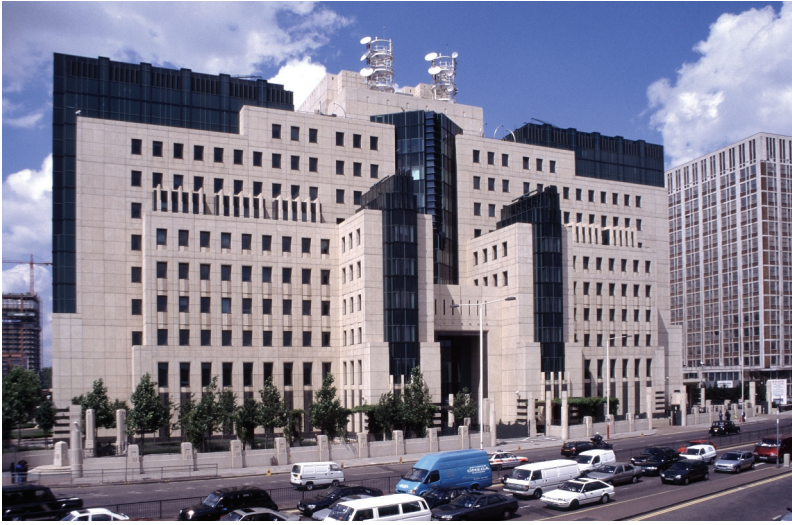
Figure 11. Photograph of the SIS Building in London, seen from the Albert Embankment. © Justin Kase RF/Alamy Stock Photo.
