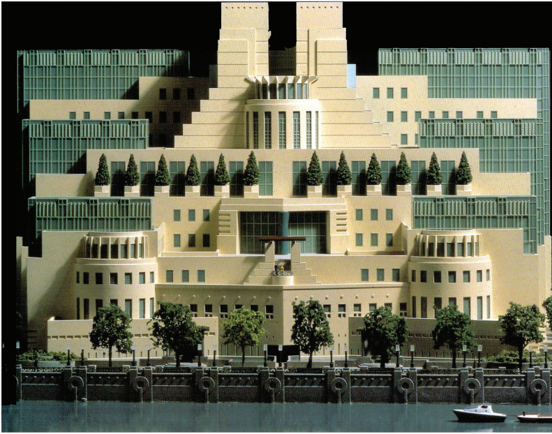
Figure 9. Scale model of Terry Farrell's final design for the SIS Building in London, circa 1988–89. The complex is composed of three longitudinal blocks with cream-coloured concrete cladding, rising in height as they move further away from the river, and linked by green glazed courtyards and atria. This photograph shows the Riverside elevation of the building. © Farrells.
