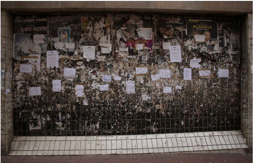
Fig. 4. Wall beneath Hillbrow Tower advertising rooms to let.
