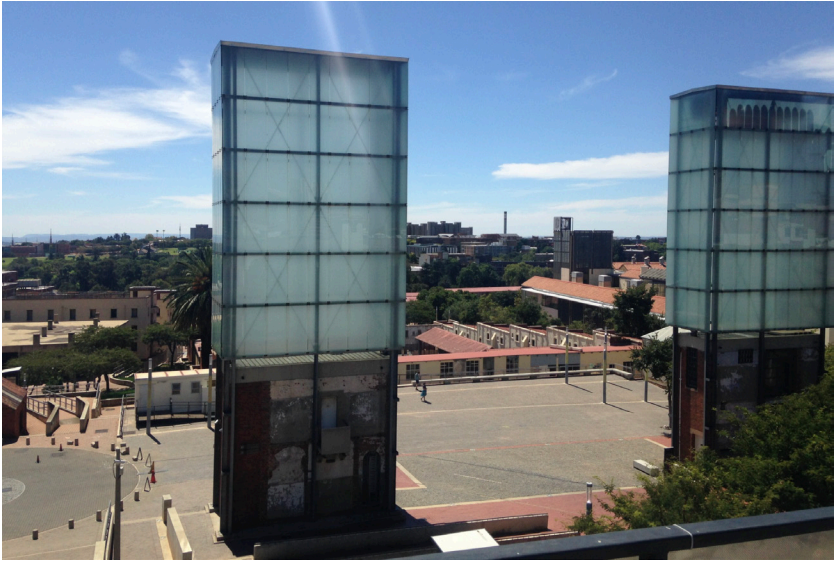
Fig. 3. The original stairwells to the Awaiting Trial Block of the prison complex, since amended with striking lightboxes.
