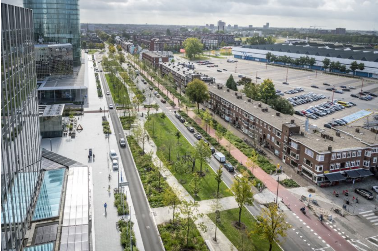
Figure 31 Croeselaan road in Utrecht
