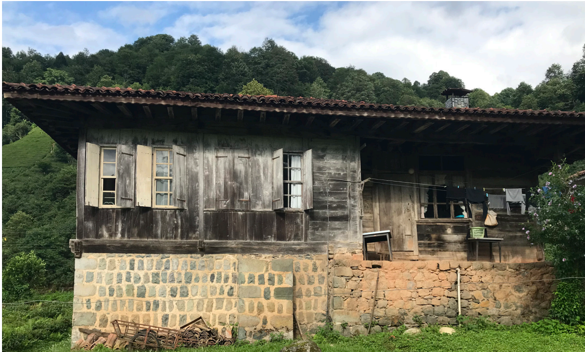
^ Fig. 2 Timber buildings elevated on stone in Hara village (Source: Gül Aktürk, Hannah Fluck, CC BY 4.0).
