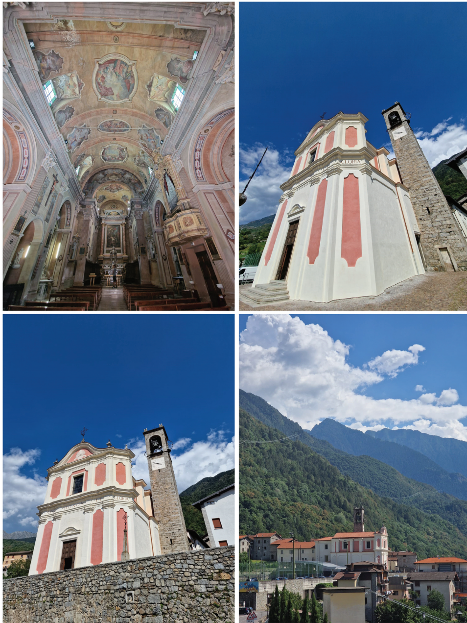
Figure 9. Views of the church of Ceto after the seismic retrofitting and restoration work.
