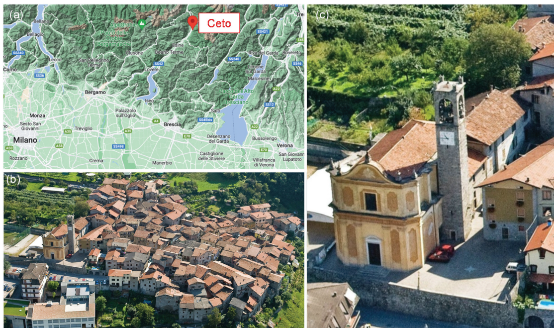
Figure 1. (a) Location of the analysed church in the province of Brescia; (b) position of the church in the town of Ceto; (c) case-study building.
