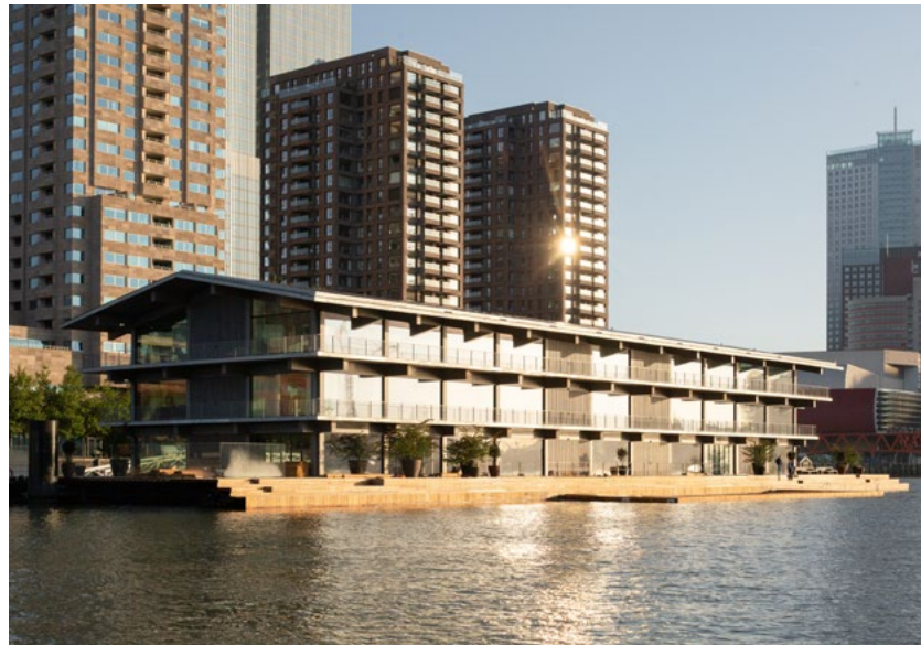
Figure 4 Where possible building on water utilizes otherwise neglected surface area and is future-proof, even with rising sea levels. The floating office featuring amongst others the Global Centre on Adaptation (design: Powerhouse Company) in the harbour of Rotterdam is the largest floating office in the world (3,600 m 2 ) (photograph by Marcel IJzerman).
