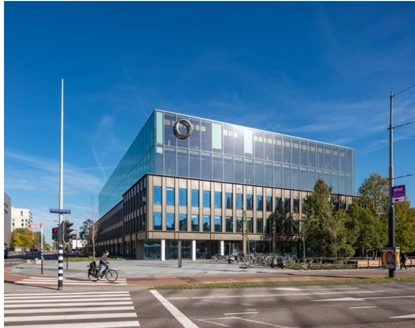
Figure 2 The Edge Olympic office building (design: Eric van Noord, de Architekten Cie.) is a successful redevelopment in Amsterdam (Well Platinum certified), where two storeys were added to the existing two-storey concrete building using a glulam post and beam construction (photograph by Ossip van Duivenbode).
